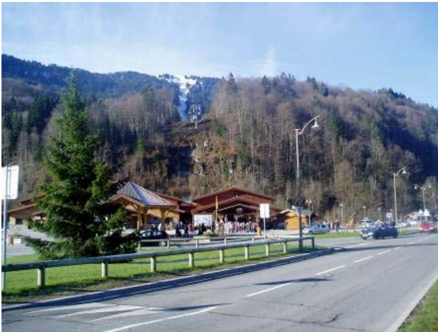
The new ski lift station
