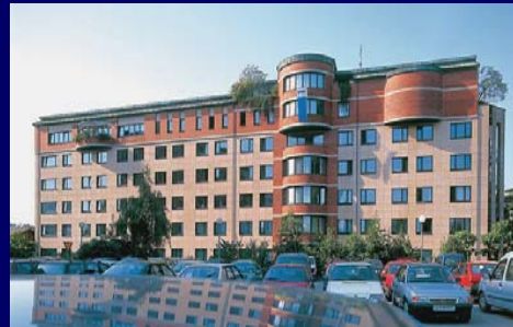
National Building and Civil Engineering Institute, Ljubljana
